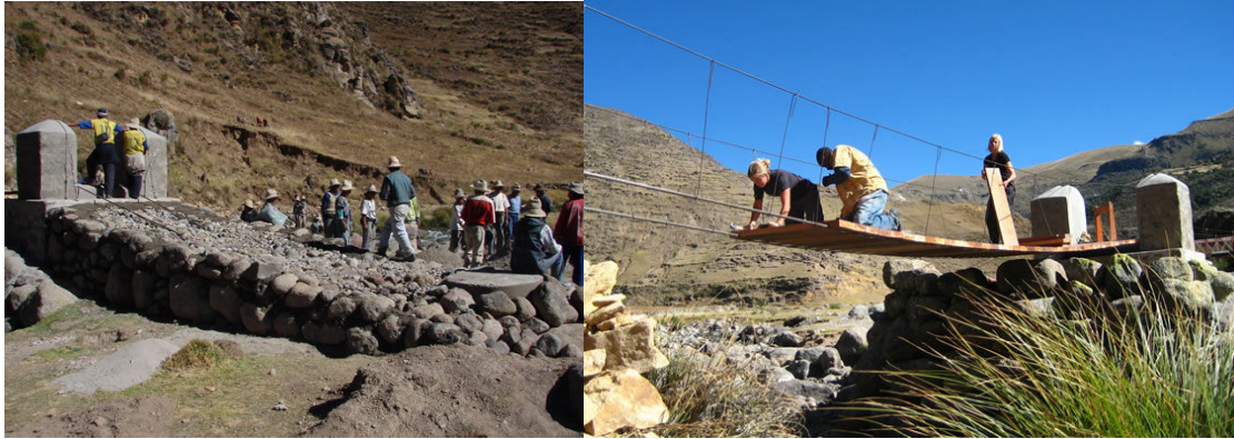
Construction of right abutment ramp
